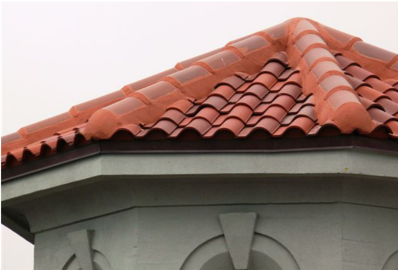
Bridge of Lions - Completed Roof - 11/24/09 #023
