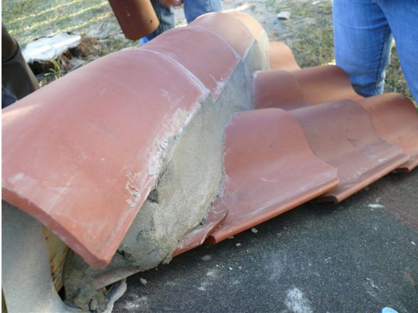
Bridge of Lions - Roof Mock-Up - 11/20/08 #005
