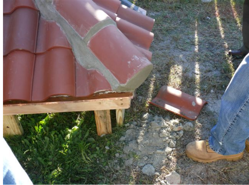
Bridge of Lions - Roof Mock-Up - 11/20/08 #006
