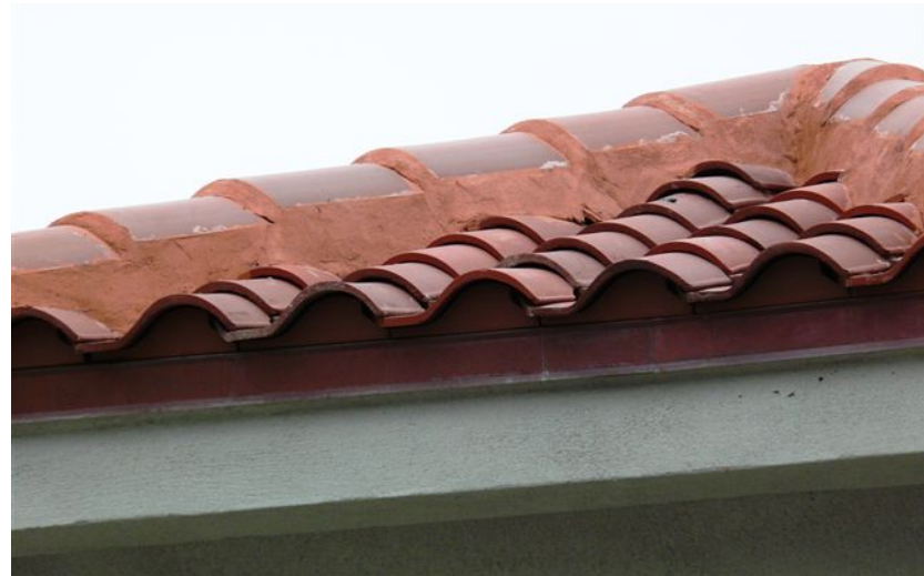
Bridge of Lions - Completed Roof - 11/24/09 #039
